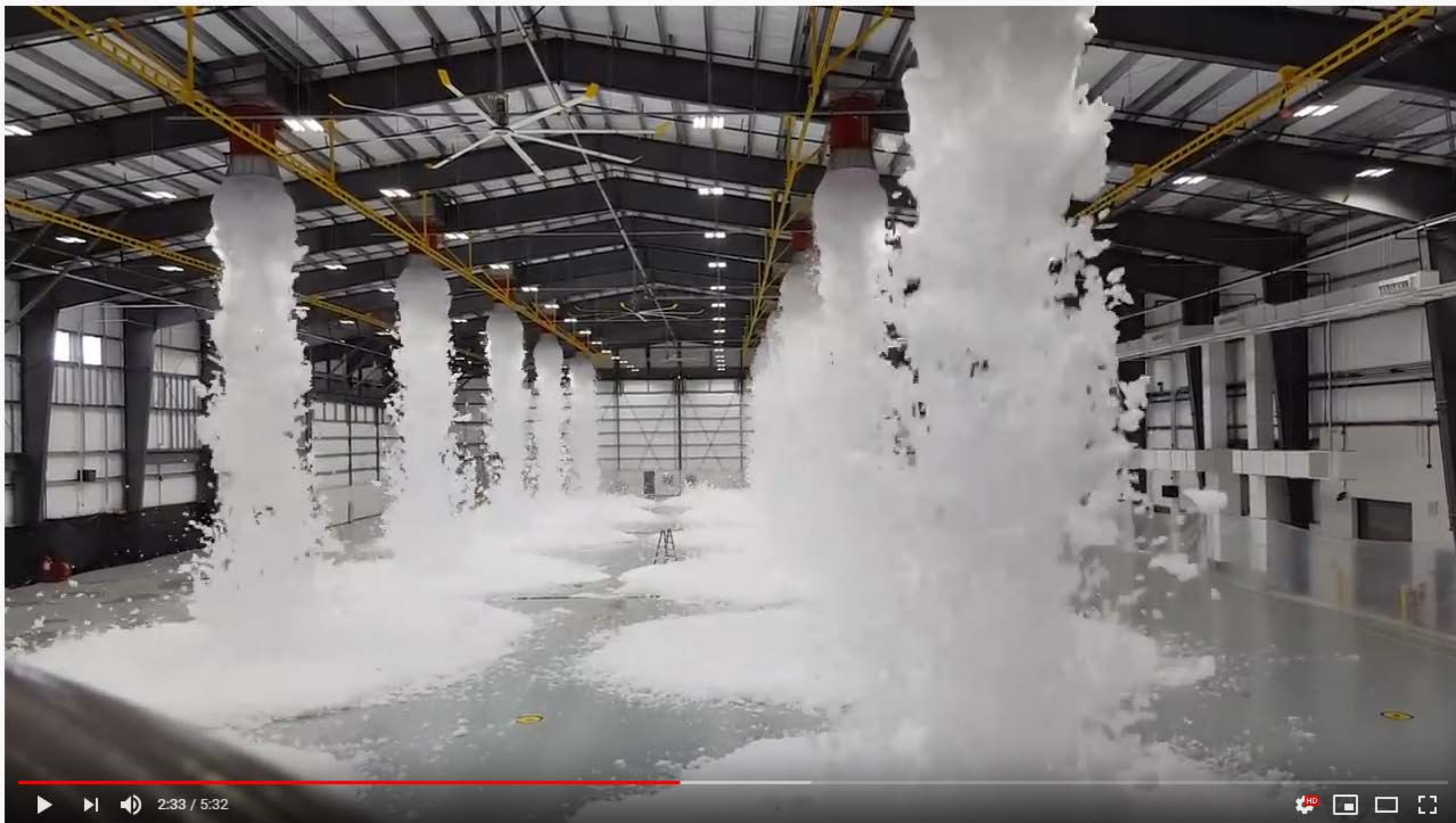
Aircraft hangar fire alarm test high expansion foam
